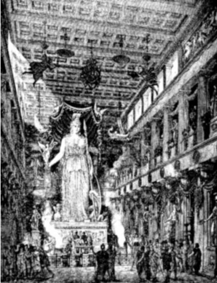
INTERIOR OF THE PARTHENON
