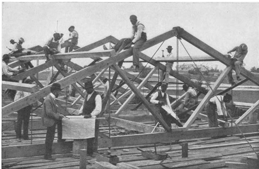
STUDENTS FRAMING THE ROOF OF A LARGE BUILDING
